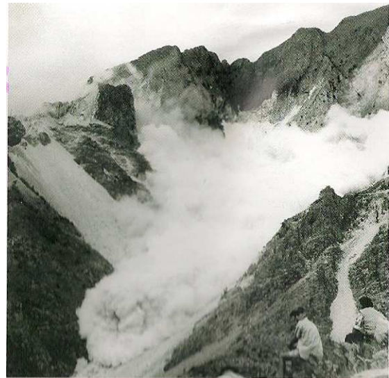
The 1932 blasting, or varata
