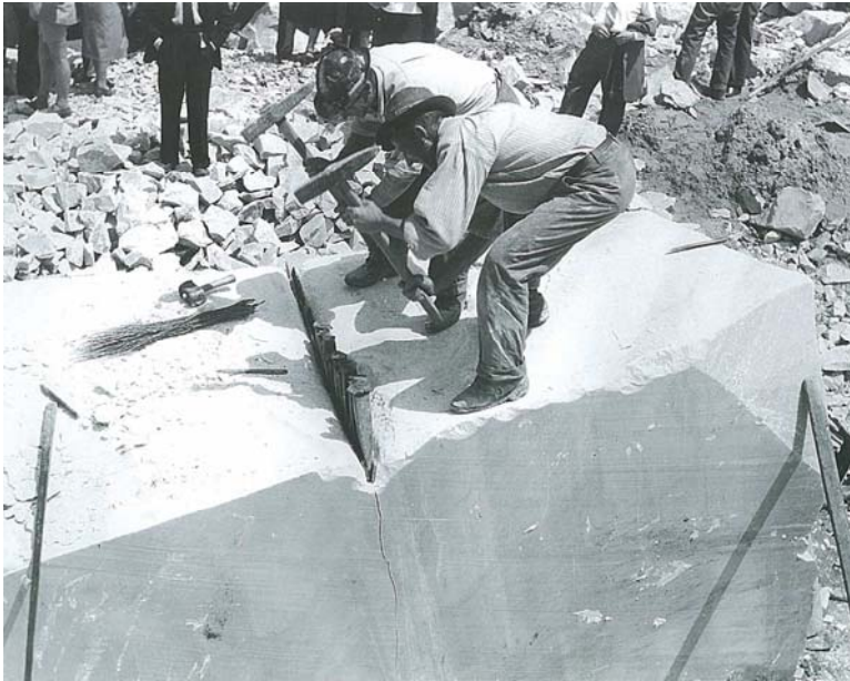
Quarrymen using the gad to cut blocks
